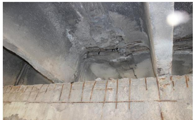
**Photo 2. Span №1. Damage to the supporting sections of the beams**
