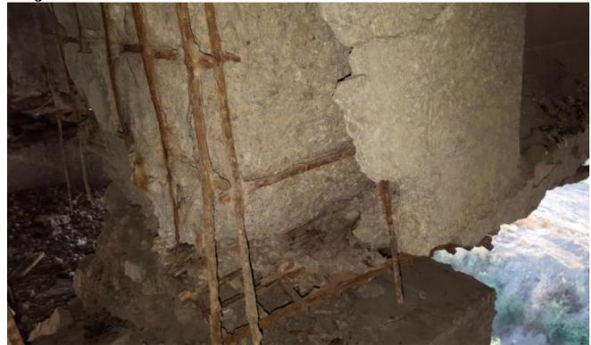
**Photo 5. Fracture of concrete and corrosion of reinforcement at the ends of beams with  $L=22.16$  m**
