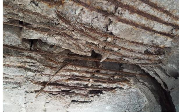
**Photo 4. Corrosion of bare reinforcement at the sites of destruction of the protective layer of concrete in the beams of the span with  $L=16.76$  m: (a) section of the beam near the drainage tube; (b) section of the slab near the expansion joint**
