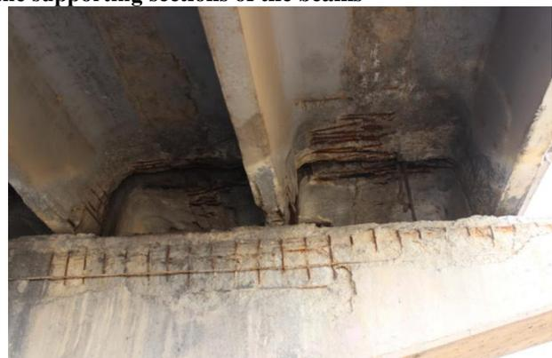
**Photo 3. Span №2. Damage to the supporting sections of the beams**
