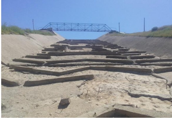
Fig 1 Damage to reservoir spillway structure caused by mudflows
