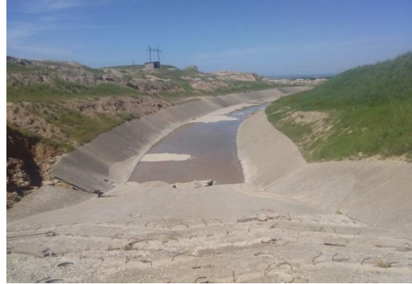
Fig 1 Damage to reservoir spillway structure caused by mudflows
