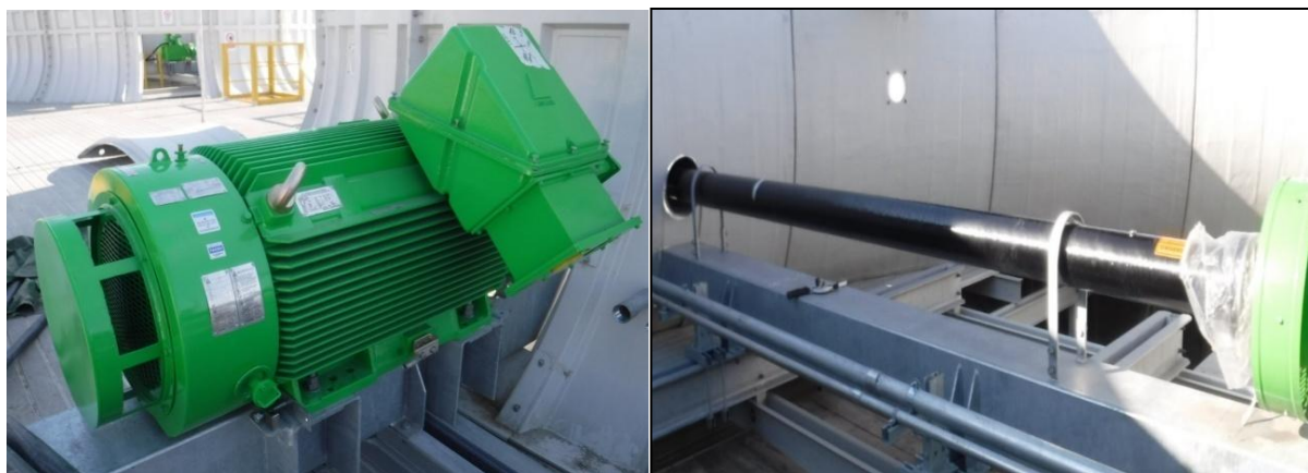
Fig. 3: Motor and drive shaft that rotates the blades.
