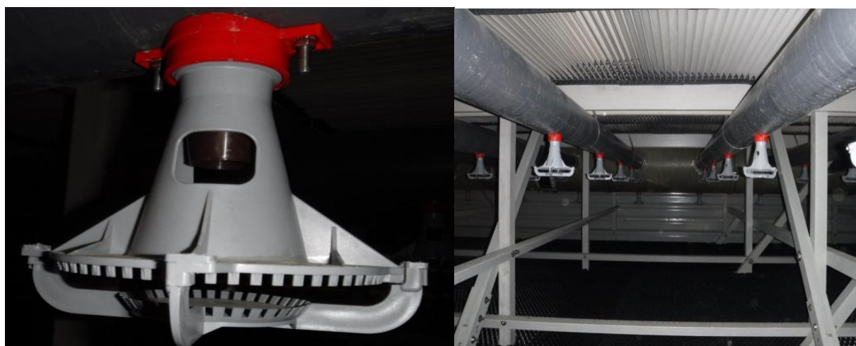
Fig. 4 Water spray nozzles.
