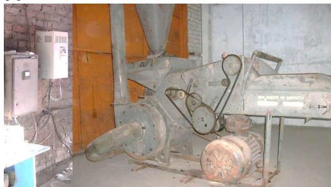
Fig.1. Control of an asynchronous motor of a universal feed chopper
