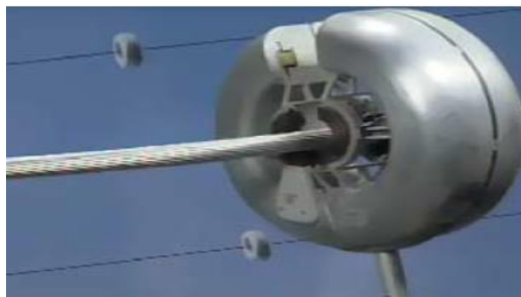
(Figure 4). Installation of the meter on the transmission conductor
