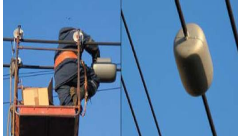
Figure 3. Installation of measuring blocks on overhead power lines.
