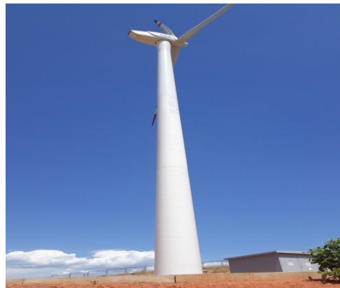
Figure 5. General view of a wind turbine 0.75 MW in the Tashkent region.
