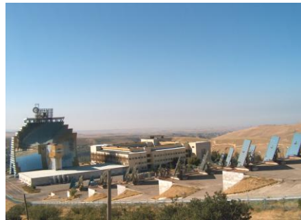
Figure 1. Big solar furnace with the power of 1000 kilowatt Scientific-industrial association "Physics-Sun" Academy of Sciences of the Republic of Uzbekistan.
