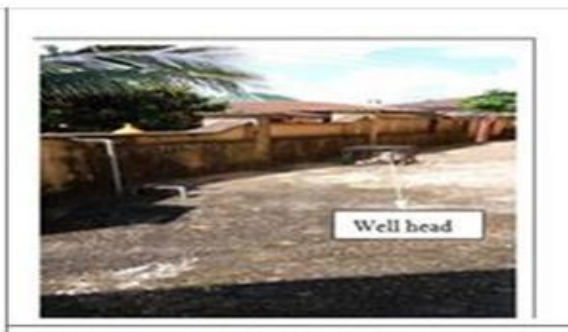
Figure 2.2: Photograph of the wellhead (inside the compound)
