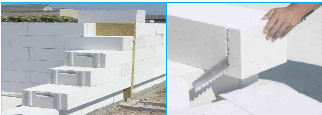
Fig4. Aerated gypsum blocks are in construction process
