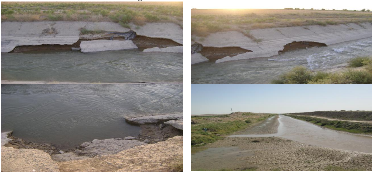
Fig.2. Technical condition of channels
