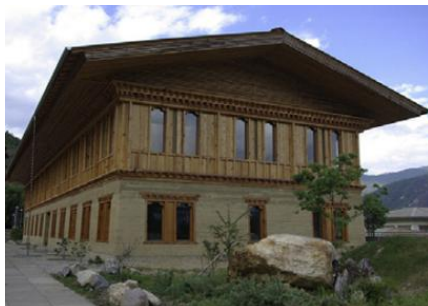
Figure 8: Building 02-University Library building, OVC
