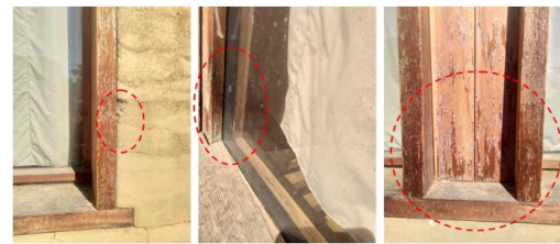
Figure 13: Typical causes of air leaks
