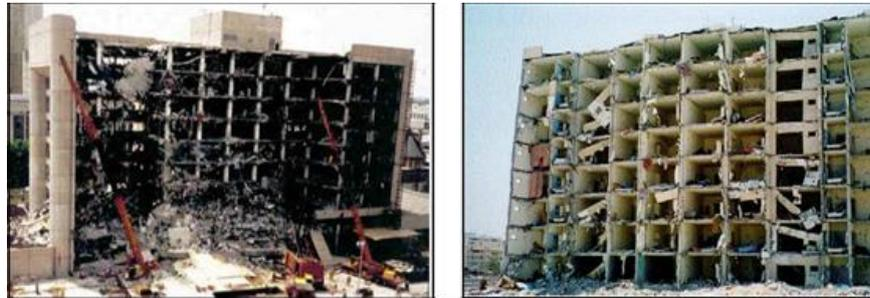
Figure 1: Effects of explosive device occurrences on buildings (Khubar Tower Figure)
