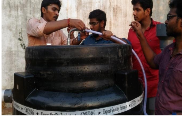
Fig.7 Gas pipeline fixing
