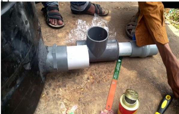
Fig.9. Emergency pipeline Installation
