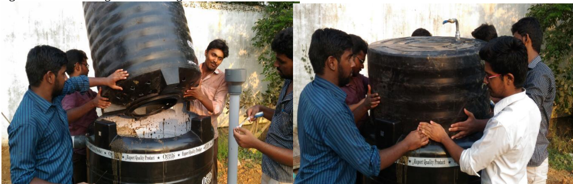
Fig.6 (a), (b) Positioning of Gas holder on Digester tank.
