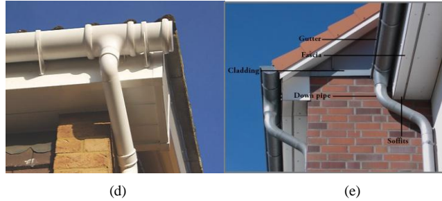
(a) Rain water Harvesting System (b) Storage of rain water (c) Basic components of rain water harvesting (d) Connecting a gutter (e) Connecting a gutter
