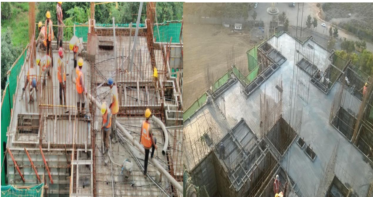
Fig.1.05. Concreting of Slab with RMC in Aluminum Formwork
