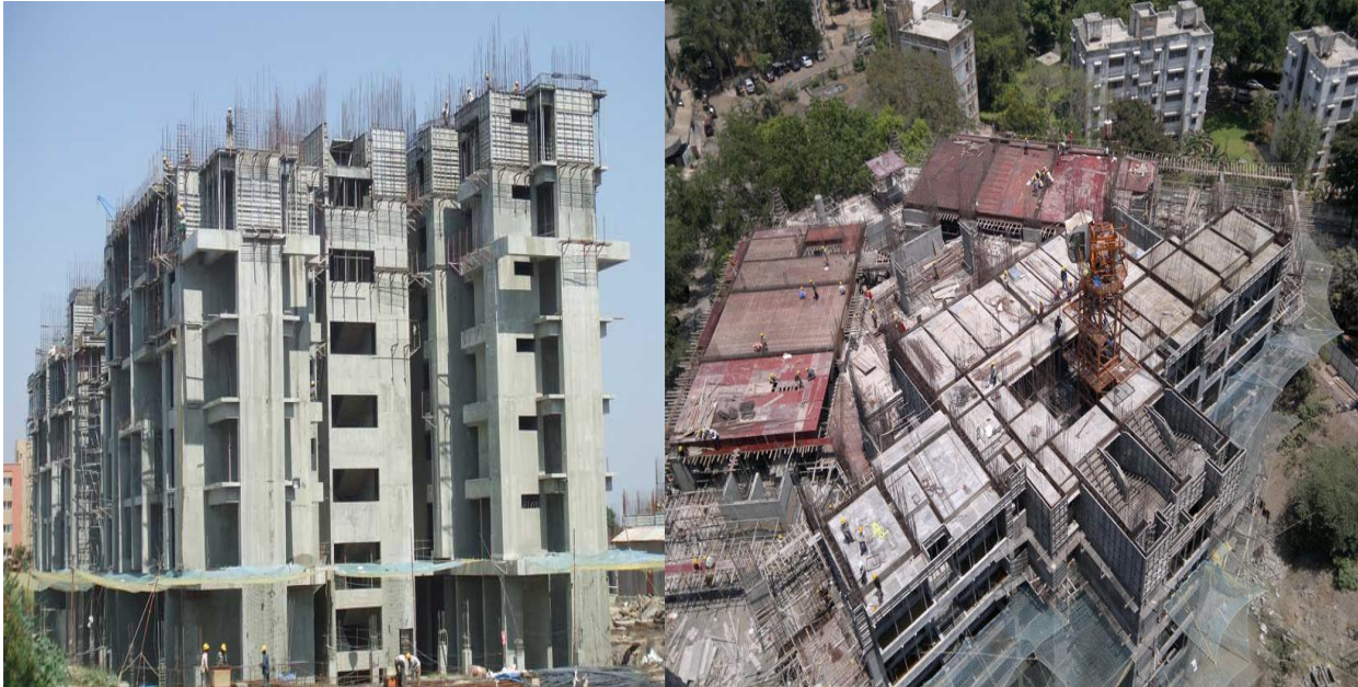
Fig 1.04.Elevation & Bird View of Aluminum Formwork Slab Construction
