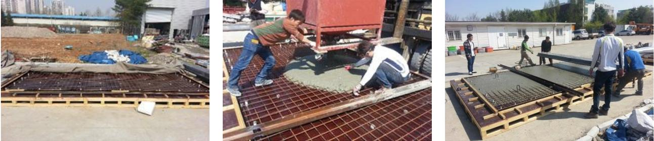
Fig. 7 Fabrication of specimen
