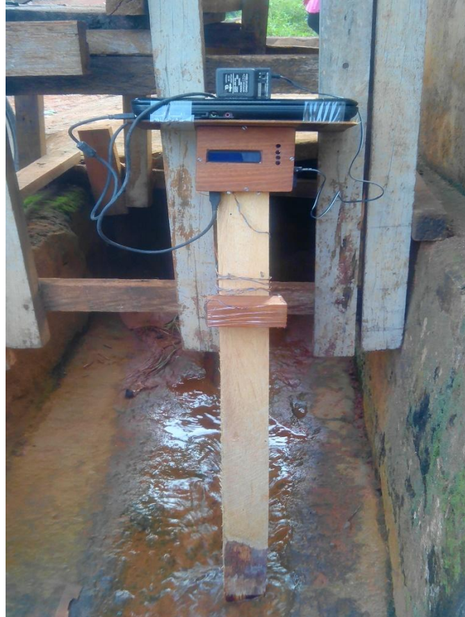
Figure 3: Installation of rangefinder in an artificial drainage system
